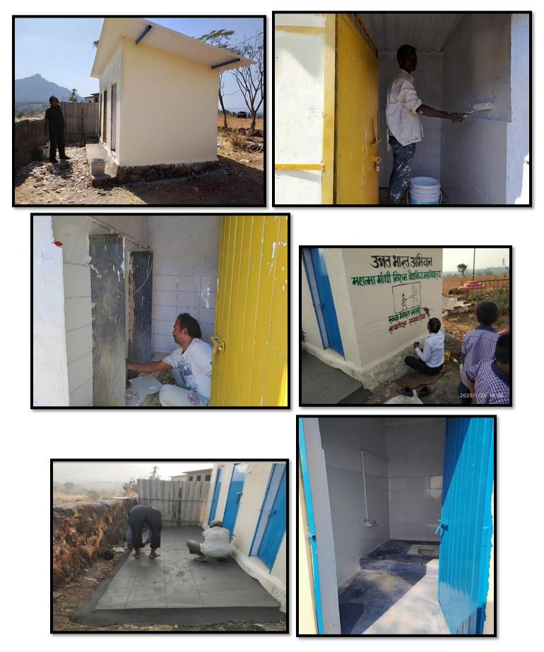
Plumbing, Water pipeline, roof construction cementing, tiling painting work conducted at school toilet blocks. Ramp has been made for accessibility.
