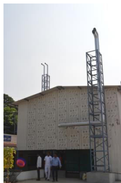
Photographs No. 1.5 DG Set with adequate Stack Height
